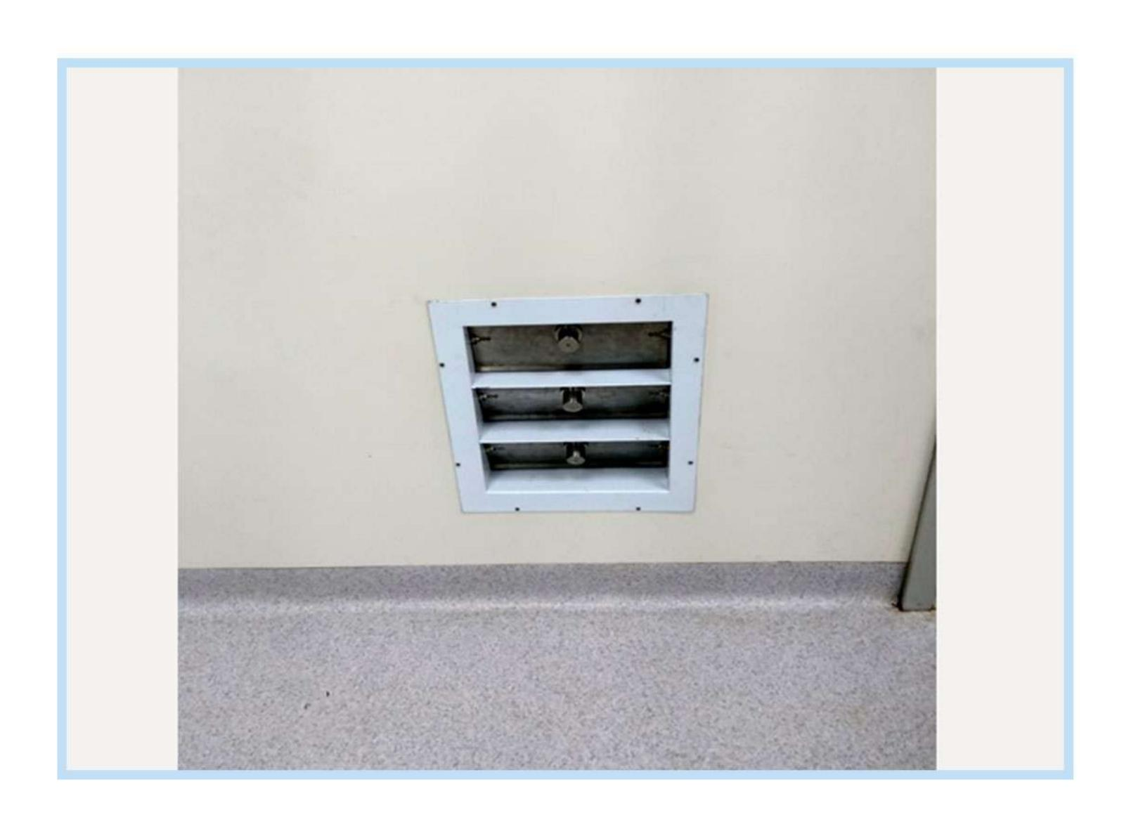
These dampers are back draft air damper that come along with the adjustable start-open pressure. These dampers are used to prevent contamination of air from clean as well as dirty areas. We offer the perfectly suitable size air pressure relief dampers and place them strategically to enable the room pressure of two different rooms when the doors are open between the dirty and clean areas.
